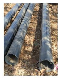
Left is a picture of the 8-inch metal pipes that were used in this new borehole. As you can see, they are much larger than the usual pipes used in most water wells. This new borehole also appears to have an abundance of water. We hit water at 70 meters (230 feet) and they ended up drilling down to 130 meters (430 feet). That should give us a lot of water!
